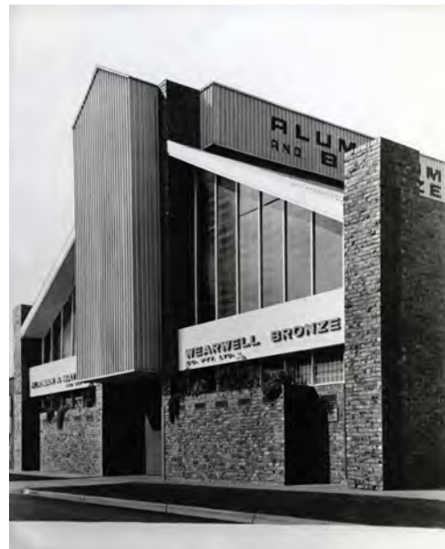
Above Factory foundry for Wearwell Bronze Pty Ltd, Northcote, Victoria, 1962 Architect, Geoffrey Woodfall, (Woodfall & Reynolds), Photographer, Lloyd Buchanan Photography, RMIT Design Archives
